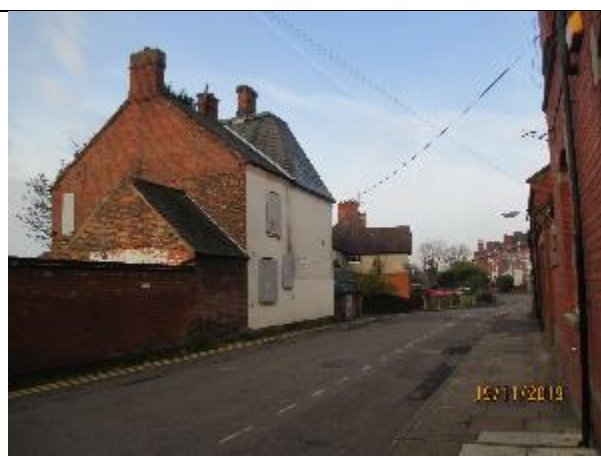
North west elevation of the Gatehouse
