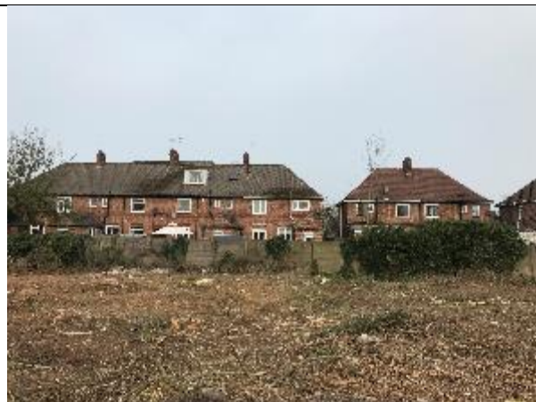
Rear of properties on Redwood Crescent, which are to the north west of the site
