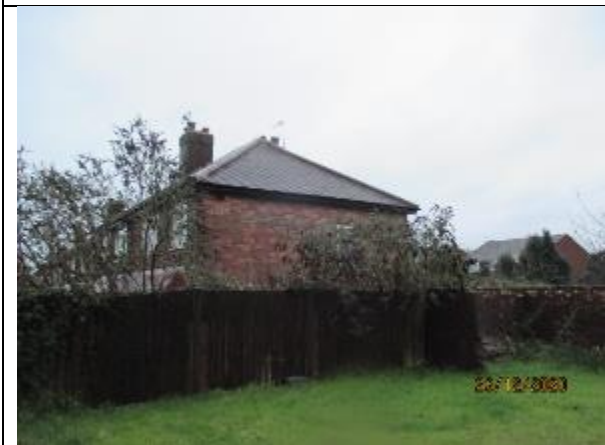
Side elevation of 23 Princess Avenue
