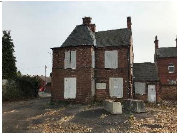
Rear (north east) elevation of the Gatehouse
