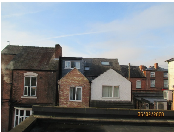
Rear elevation of 5, 3 and 1 City Road (l to r)
