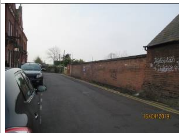
Existing boundary wall to the site
