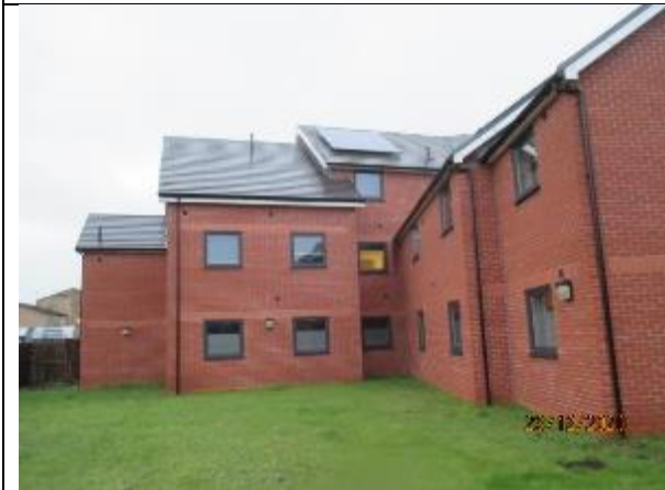
Rear (south east) elevation of Flewitt House
