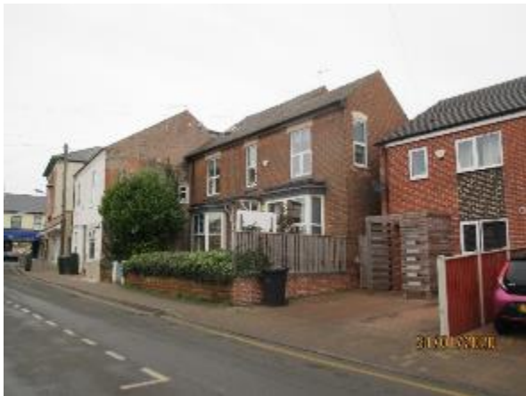
Front elevation. 7 City Road is to the right, with 1 and 3 City Road to the left
