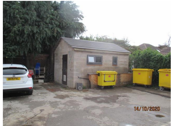
Outbuilding, located in the western corner of the site
